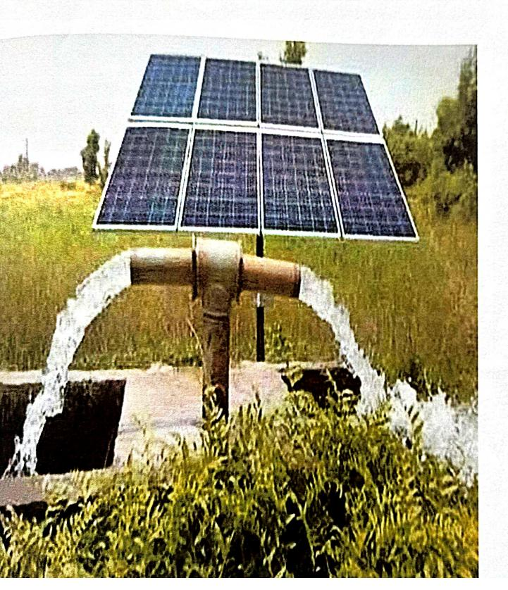
In solar pumping, the power generated by solar-energy is utilized for pumping water for irrigation purposes. The requirement for water pumping is greatest in the hot summer months which coincide with the increased solar radiations during this period and so this method is most appropriate for irrigation purpose. During periods of inclement weather when solar radiations are low then the requirement for water pumping is also relatively less as the transpiration losses from the crops are also low.
